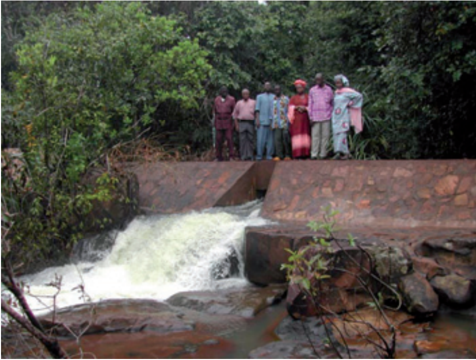
Sirakorobougou (Mali): Dam
